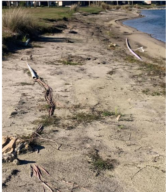
Damaged Irrigation Lines #7 Tee Box
